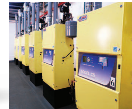
MULTI BOILER ARRAY
