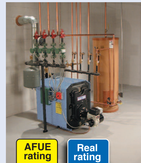
Typical high-mass boiler with indirect water heater.
